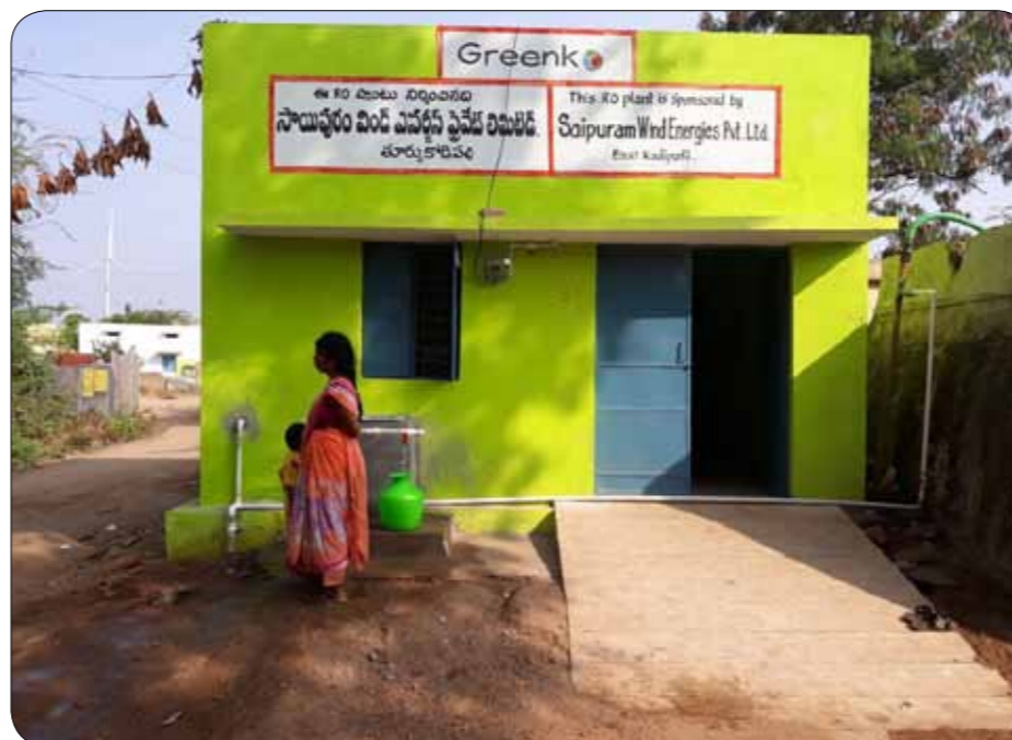
RO Plant installed at East Kodipalli
