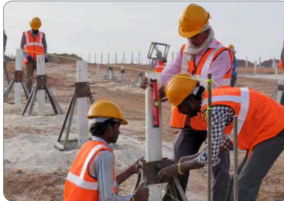
Solar Project Execution
